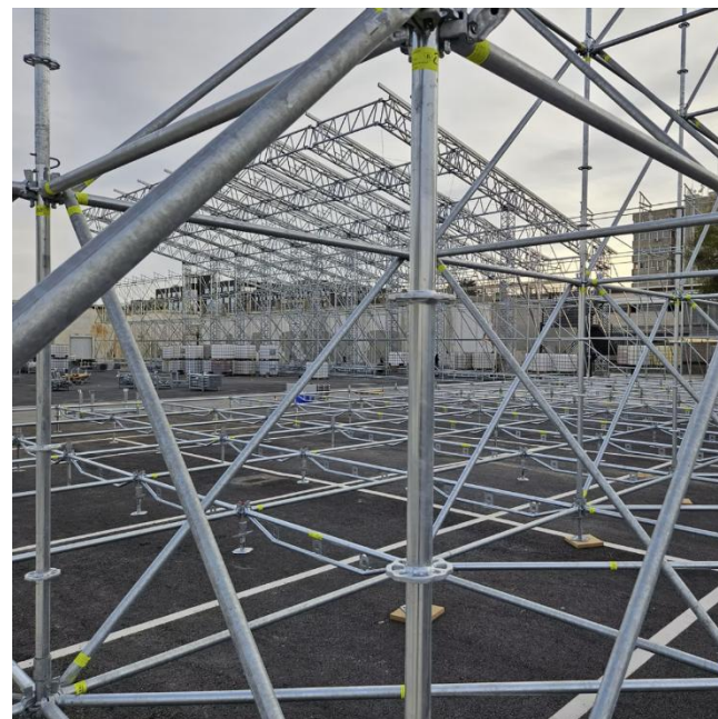
Pavillion of scaffolding and COVEX roof
